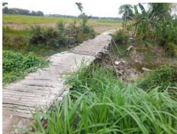
Figure 1. Existing Condition of Sroyo Village Bridge
