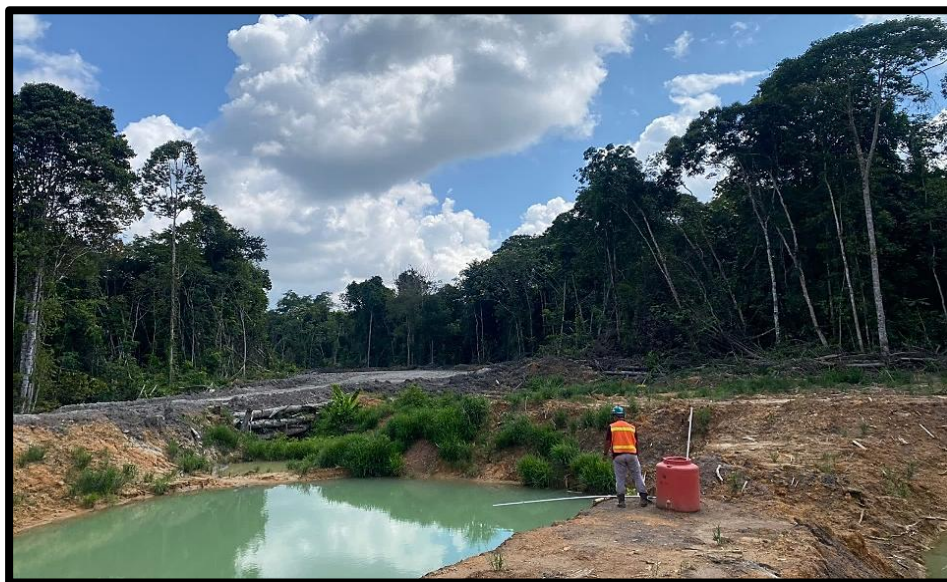
Figure 3. Settling pond area
