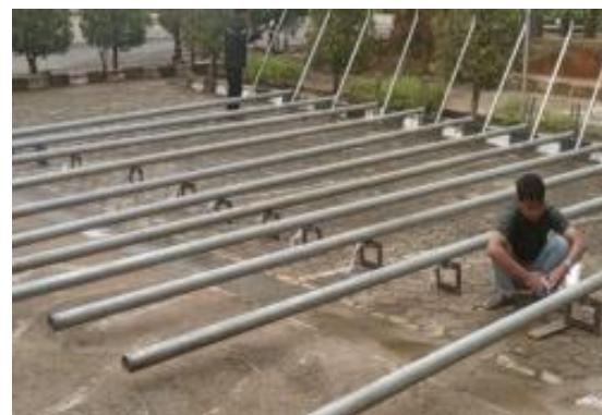
Gambar 6. Finishing tiang PJU
