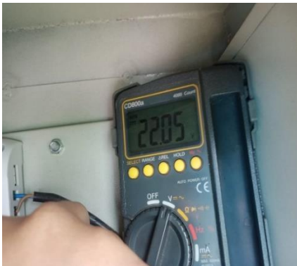
Gambar 11. Pengukuran Langsung Voltase Panel Surya
