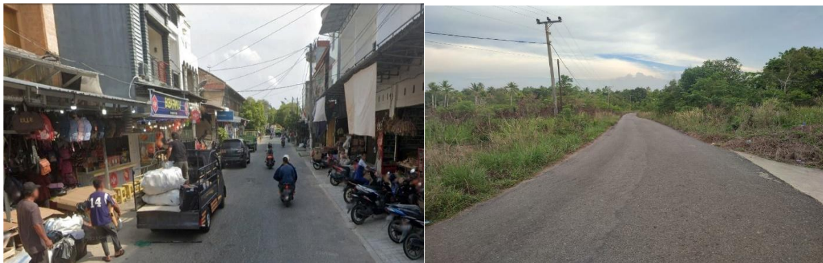
Figure 3. Existing condition of the road network in West Bangka Regency
