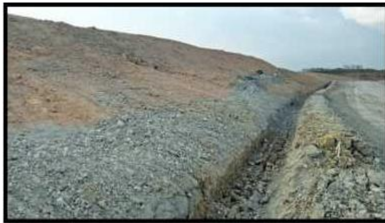
Figure 5. Drainage Channel Manufacturing
