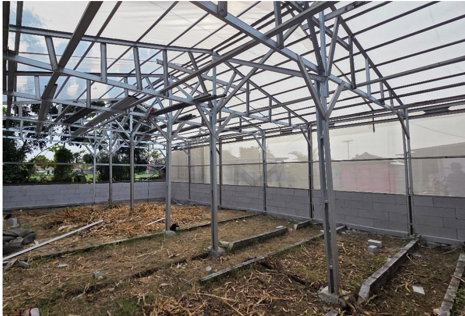
Figure 3. Ongoing installation of lightweight steel structures for the greenhouse.
