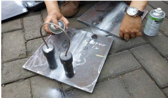
Gambar 12 Proses magnetizing test pengelasan repair 1x
